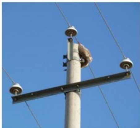
Afbeelding 3,4: Pylon with centre top pins and dead Saker, Mongolia (photo A. Dixon) and retrofitted, safe for
